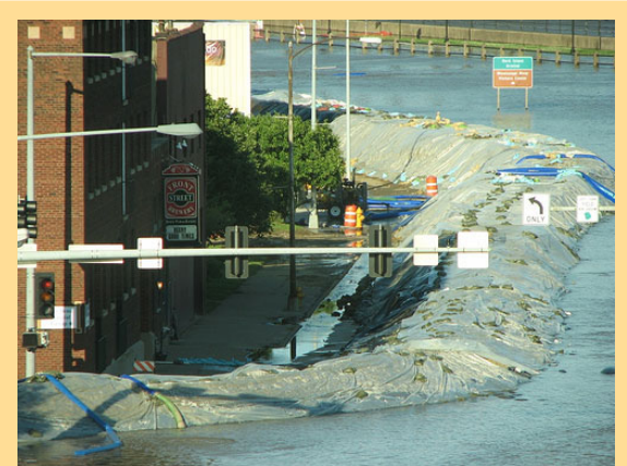
Save the beer! Temporary levees like this one protect older businesses including the Front Street Brewery
