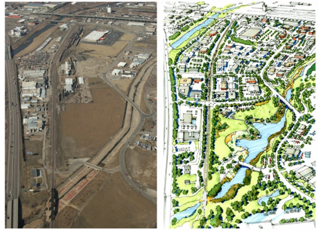
Before and after of the Sandpoint and Sioux Creek Old High Channel.
